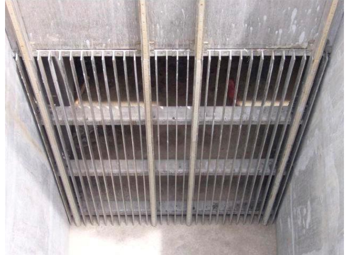
Figure 1: Coarse bar screen for wastewater treatment. Water flows through collecting large debris. Screens range from 6 - 150mm [2] [3]
