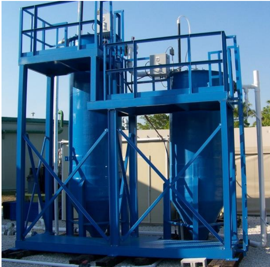
Figure 49: Hybrid depth filtration unit installed in the field
