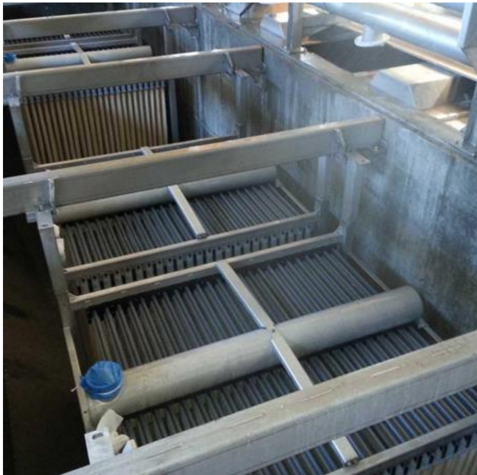
Figure 38: Image of Xylem Membrane Bioreactor showing membranes
