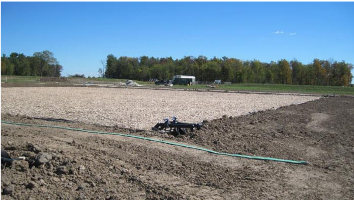
Figure 21: Completed SAGR bed topped with mulch [21]
