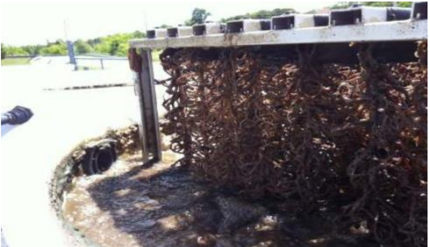
Figure 25: Solid material collected by the BioCord substrate contained in a tank
