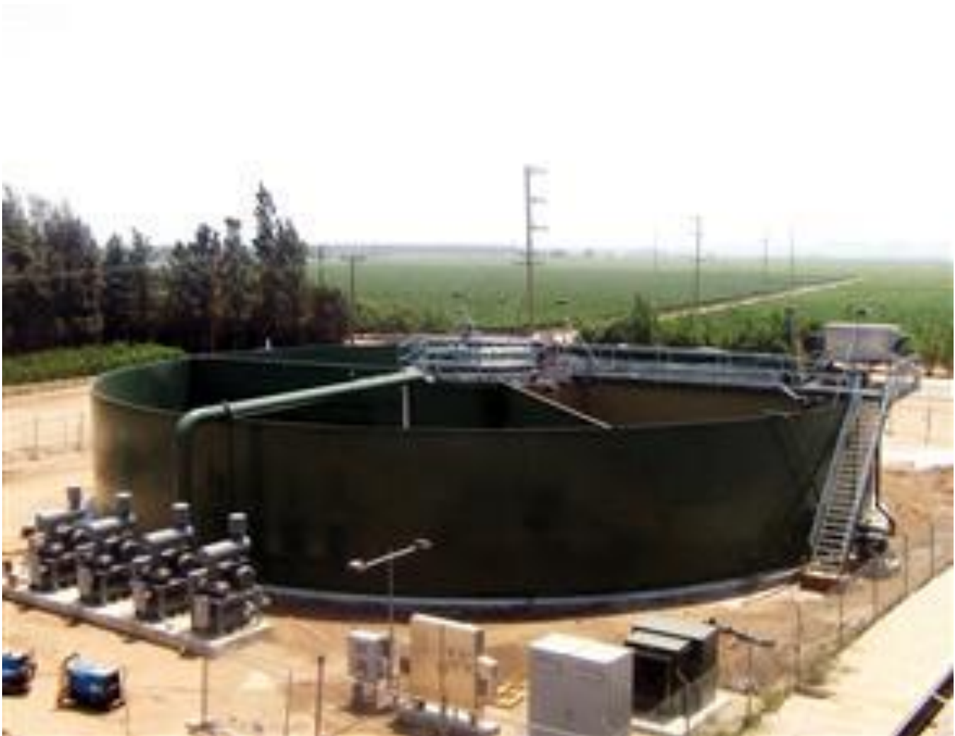
Figure 39: Titan membrane bioreactor in the field
