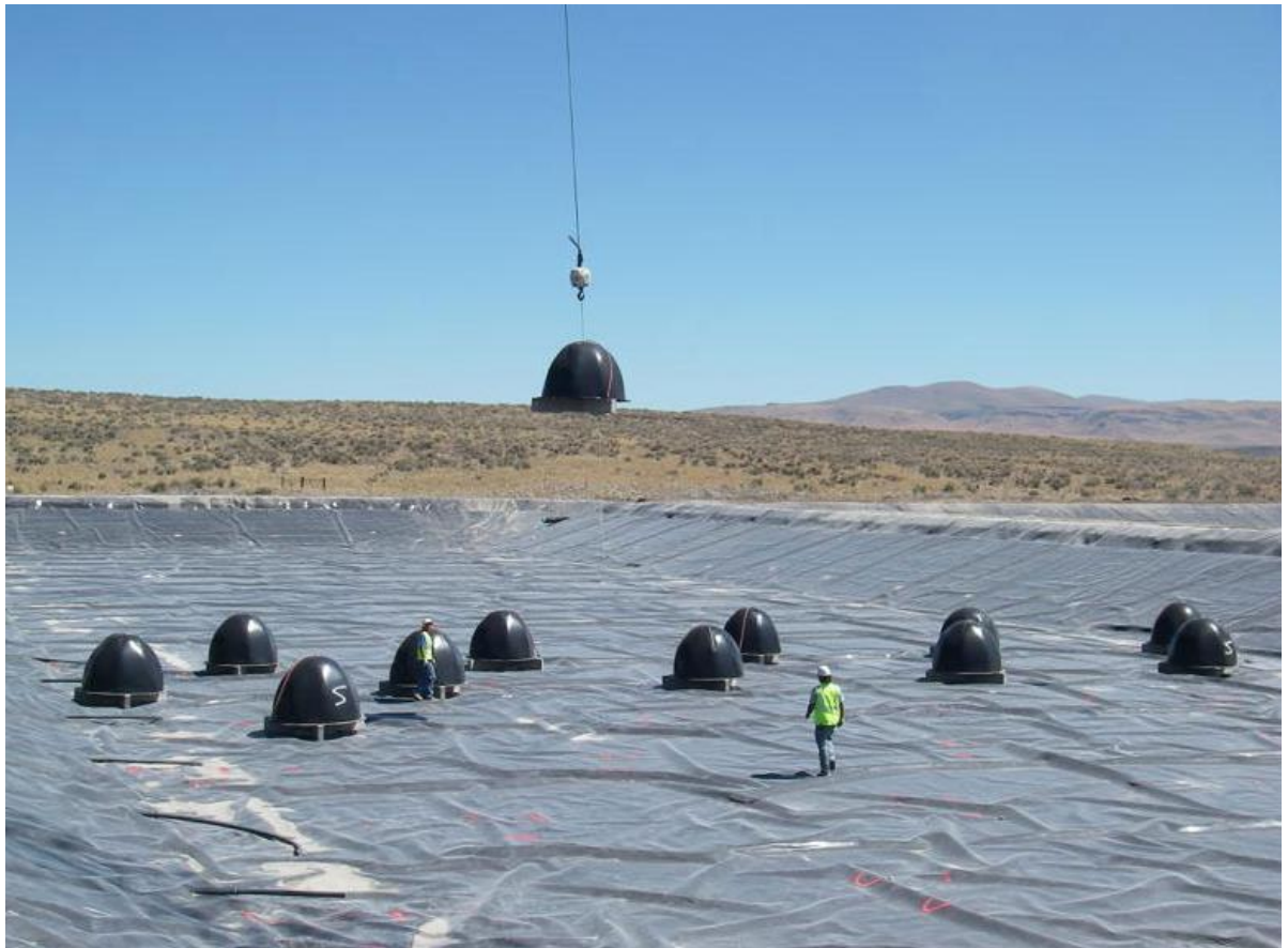
Figure 13: Bio-Domes being installed in a lagoon with a crane [17]
